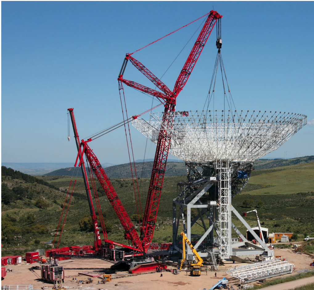
Fig. 5. The picture was taken during a crucial day for the SRT project (22 May 2010) when the structure hosting the primary mirror of the telescope was lifted on top of the alidade. That required to enroll the tallest crane available in Europe (above 100 meter in height), here depicted in red. A similar operation had never been attempted before at any other 64m (or larger) radio telescope, but Nichi D'Amico, although conscious of the putative risks, explicitly pushed for that. Everything went fine and this operation saved at least 1 year to the total construction time of the telescope (credits: INAF-OAC).
